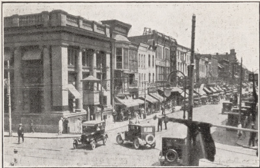
Main Corner, looking East on Dundas St.
