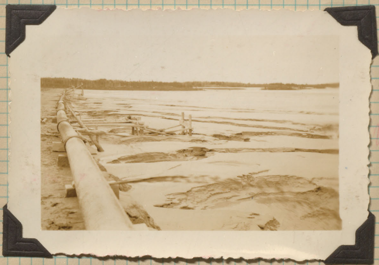
Method of Spraying Slimes
