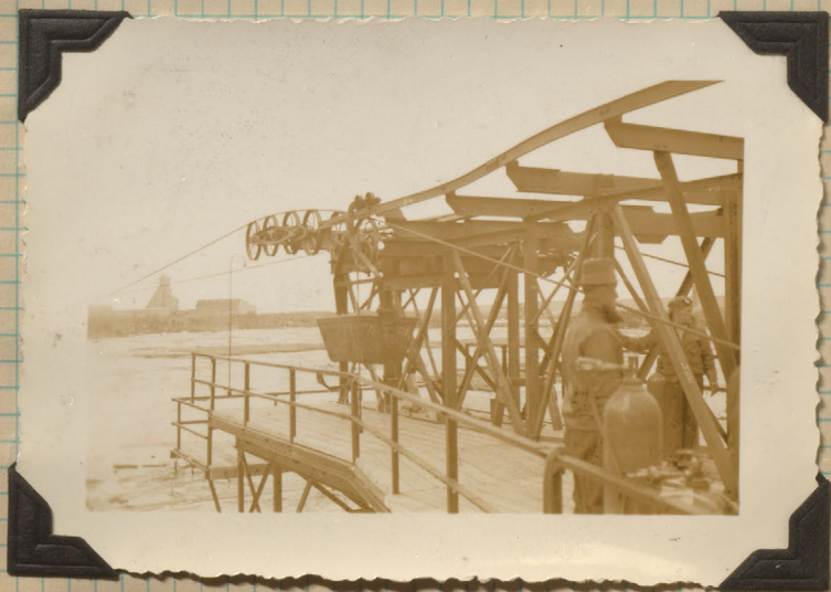
McIntyre Take off conveyor
