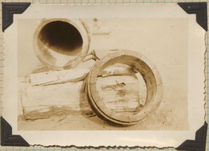
(Tailing Dam). 12 in. diam pipe. Wood Stave Pipe & Coupling - Used
