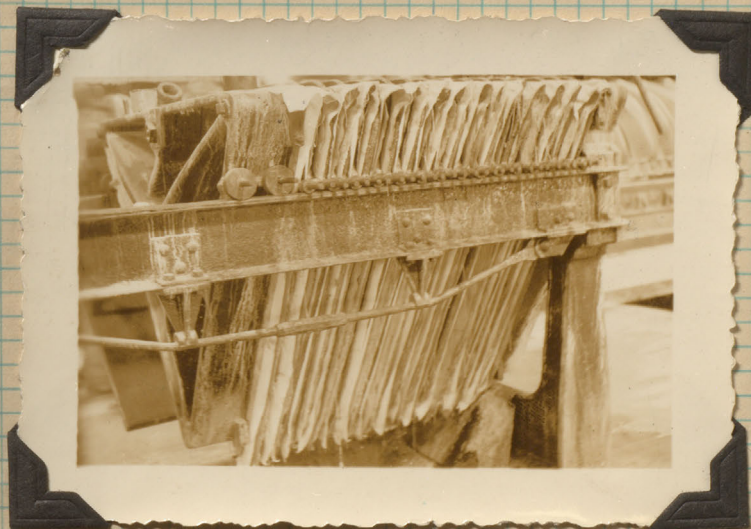
Merrill Triangular precipitation Press .
