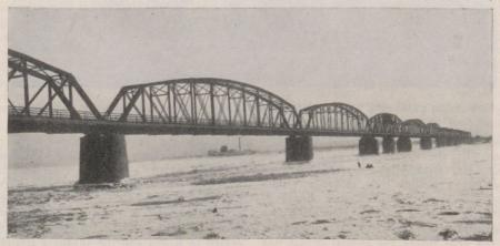
Fig. 13 represents the railway bridge over the Yalu River between Manchuria and Korea—evidently a pin-connected structure and, therefore, not quite up to the latest American practice April, 1930.
