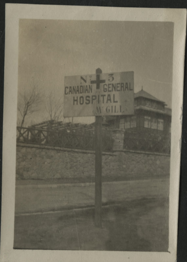
The road to our main entrance gate. No 3 CGH.
