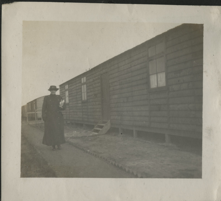
The Huts in our lines at Boulogne
