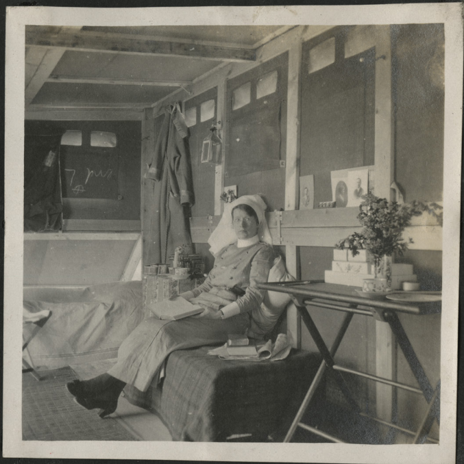
The Interior of the Armstrong Hut
