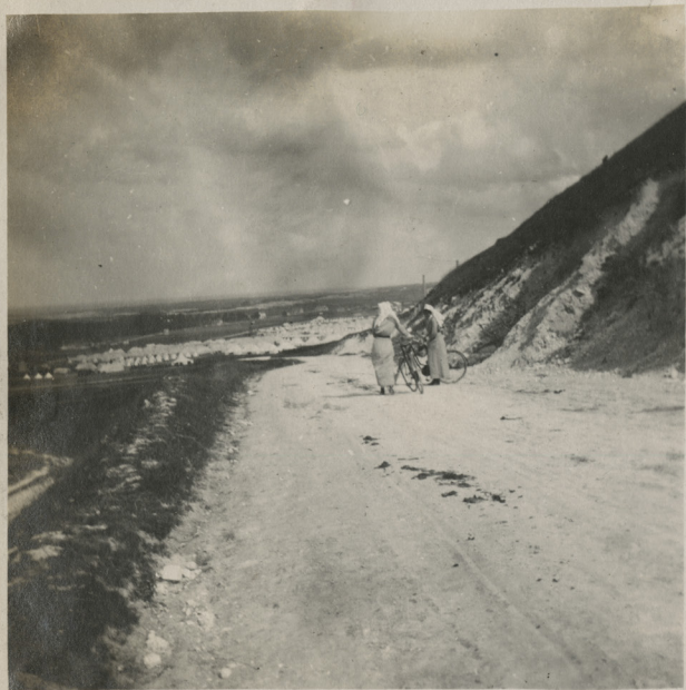
On the road above Camiers
