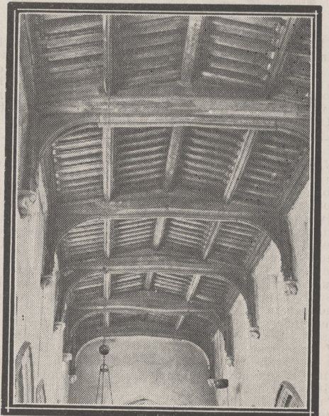
A portion of the roof showing fine scantling and wonderful preservation. The double tie beam referred to in the text is seen in the foreground. (From a photograph by Mr. F. E. Howard.)
