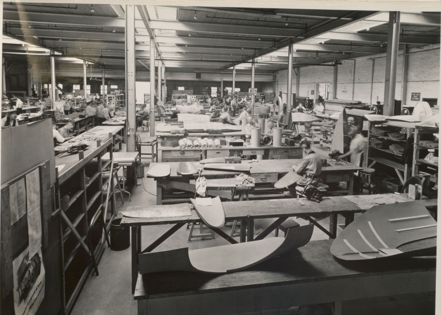
TAD 34 - C.C. & F. Co. Ltd. - AIRCRAFT DIVISION :- FORMING DEPT. - PARTS FOR FAIREY BATTLE, ANSON CARBURETTORS, CONSOLIDATED OXYGEN BOTTLES CONTAINERS, ETC.
