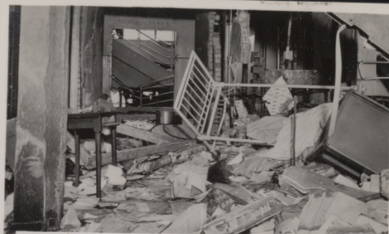
ONE OF THE WARDS OF THE HOSPITAL FOR SICK CHILDREN, GREAT ORMOND STREET, LONDON, W.C.1., DAMAGED BY A H.E. BOMB. OVER £50,000 WORTH OF DEVASTATION WAS CAUSED.
