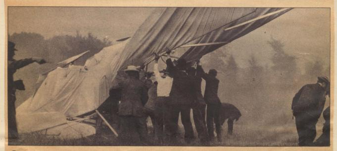
**6** Suddenly the Plane Crashes. Men at the right are clustered about Selfridge. Others are removing Wright, who is still in the plane. After circling the field three times, the ship was thrown into a dive when a tail wire snapped, fouling and breaking off the left propeller.
