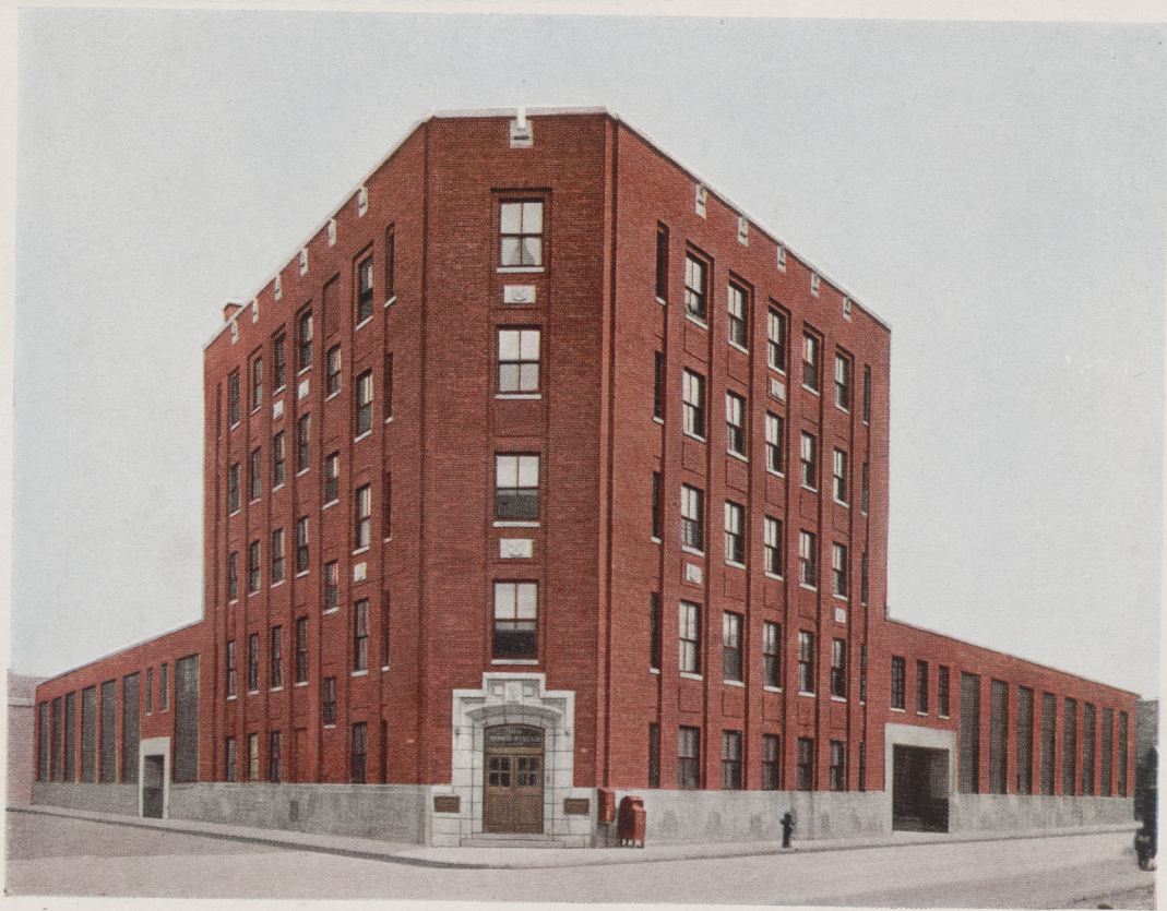
Factory in Montreal, built of Laprairie "Plastic" Brick
