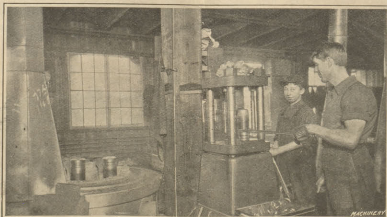
Fig. 27. Closing in Nose of Shrapnel Shell in Hydraulic Press
