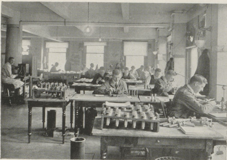
Fig. 107. I.M.B. Gauge Inspection Office, Ottawa.
