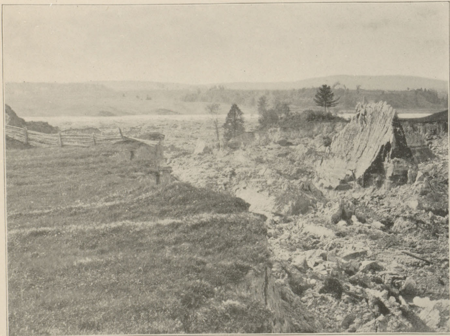
FIGURE 2.—OUTLET OF LANDSLIP, LOOKING TOWARD BLANCHE VALLEY
