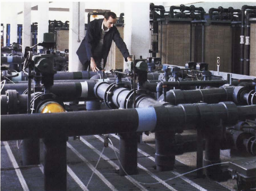
Ionics, Incorporated, a company in which Textron's American Research and Development Division has an investment, designed and constructed the demineralization plant to provide fresh water for the municipality of Corfu on one of the main tourist islands of Greece. Ionics is one of the world's leading producers of water purification and desalination equipment. Here an engineer checks the pipeline leading to special membrane stacks where brackish water is purified by transfer of salts through electrically conductive membranes.
