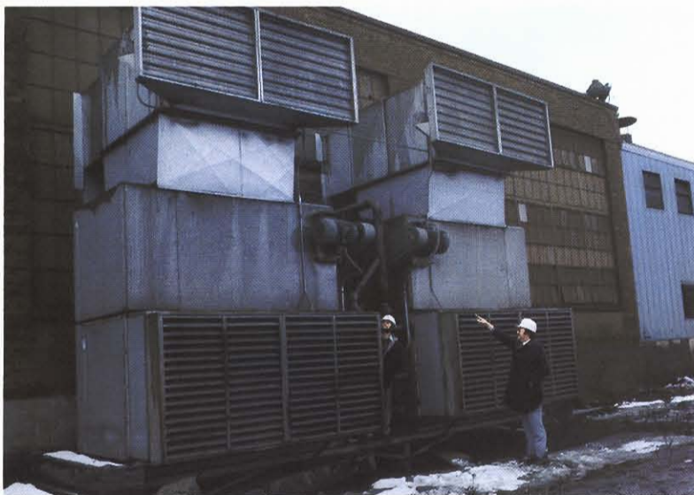
Large heat exchangers at CWC Castings save energy by utilizing the heat from oil used in manufacturing processes to warm outside air for interior area heating. The CWC exchangers are saving approximately $17,000 a year in energy costs.
