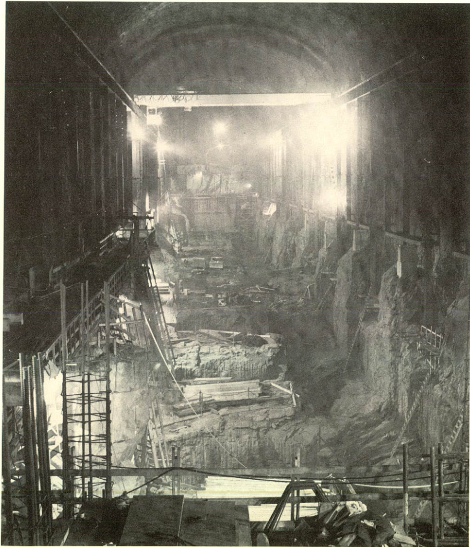
Powerhouse Excavation
