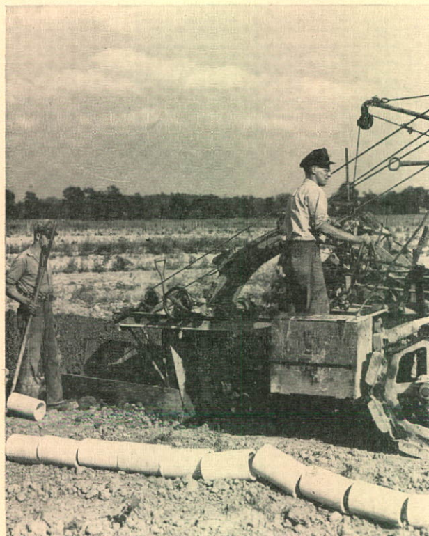
Soil management is an important factor in Bright's success in growing special wine grapes. Here new drainage is being put in to ensure the proper moisture control.
