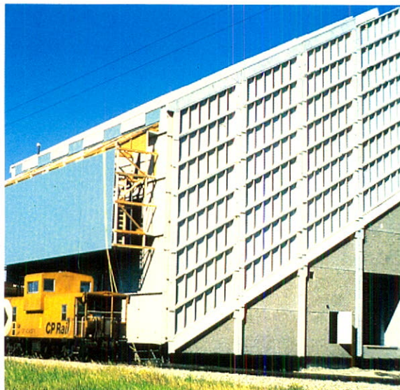
Magrath sloped bin precast concrete elevator under construction.
