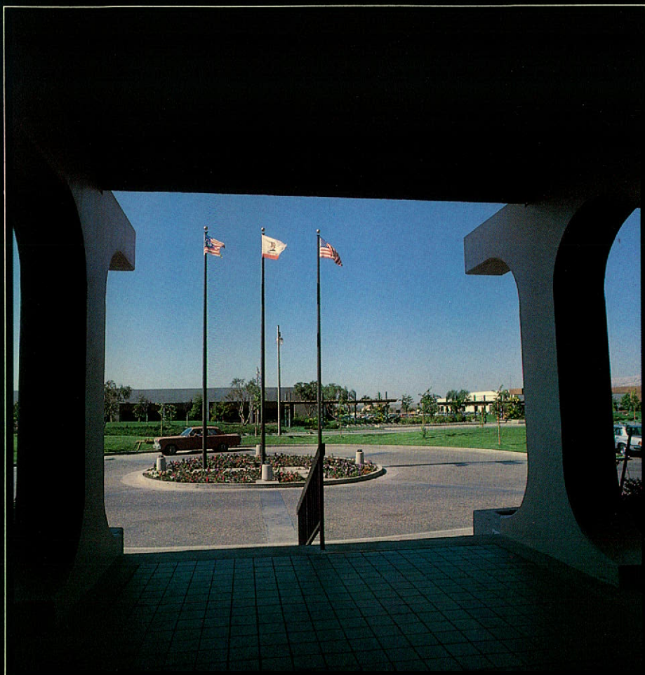
Industrial Park / Parc Industriel, Oakmead, California
