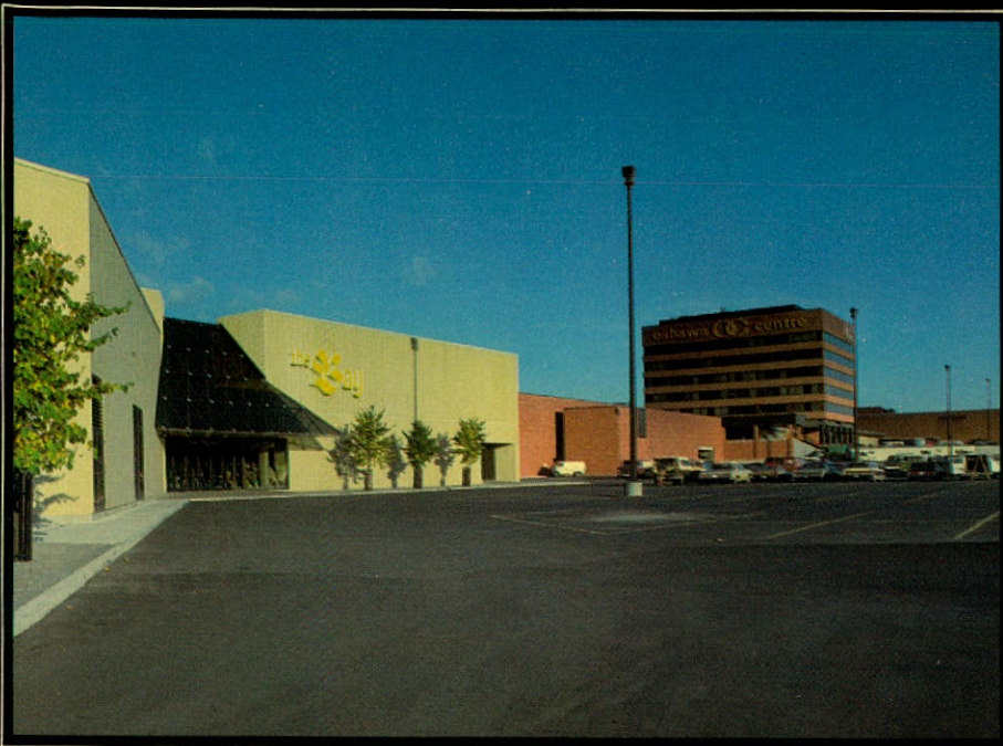
Centre commercial Oshawa / Oshawa Centre, Oshawa, Ontario
