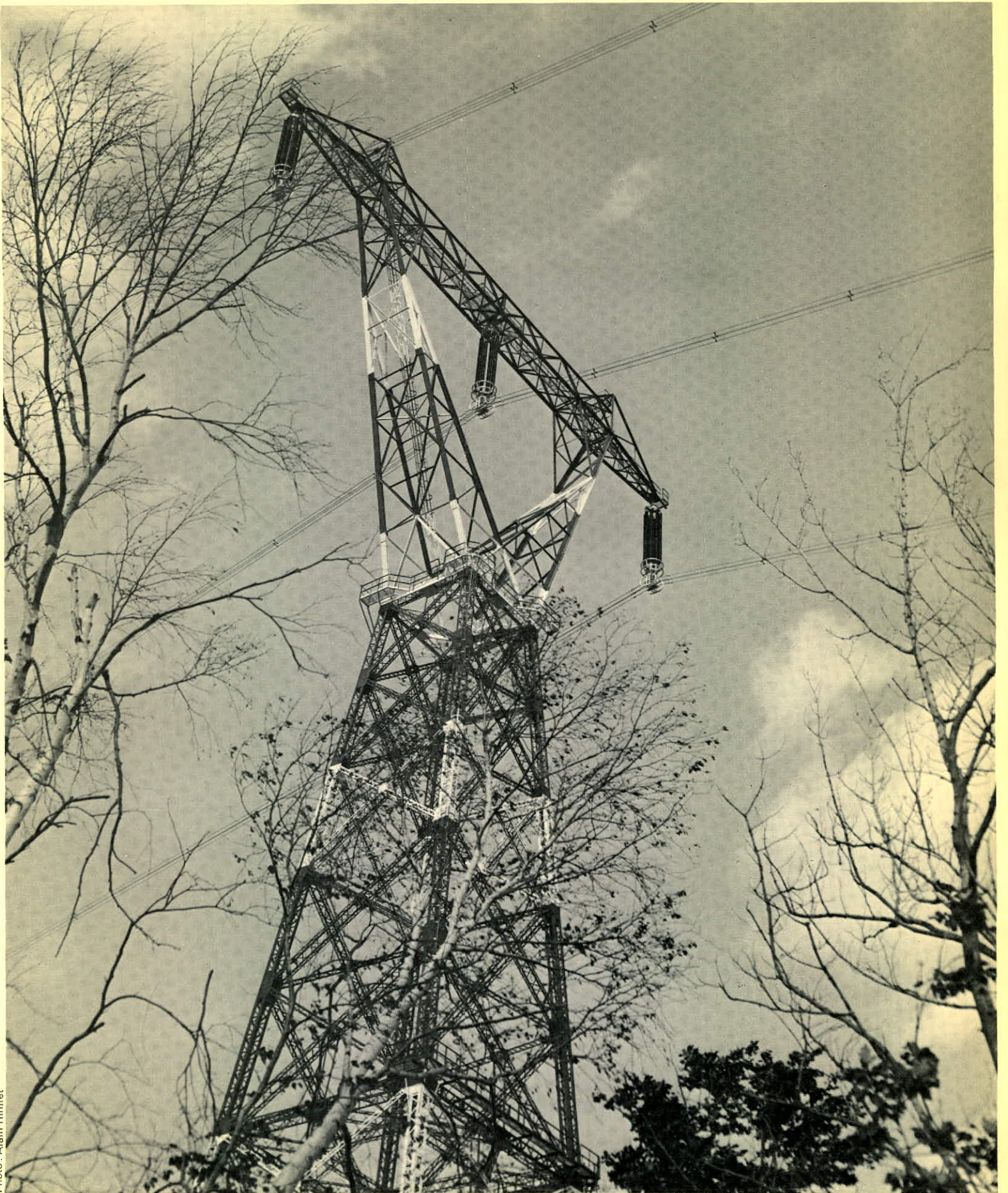
735-kV suspension tower near Quebec bridge.
