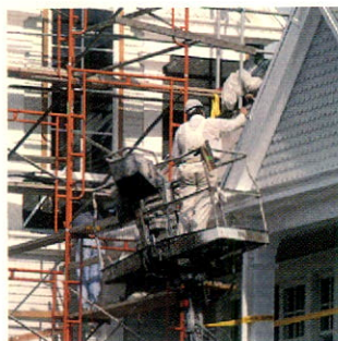
A painter enameles trim on the roofline at the Disney Yacht Club Hotel, which will open in the fall.
