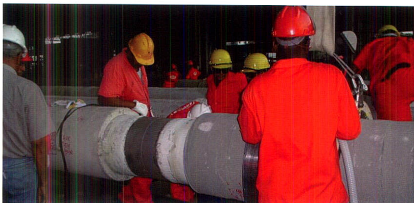
Advanced polypropylene joint protection systems for offshore pipelines
