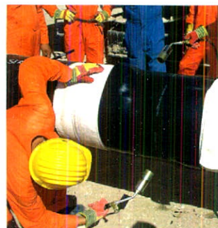
Field application of Canusa-CPS GTS-PP heat shrinkable sleeves in Kazakhstan.
