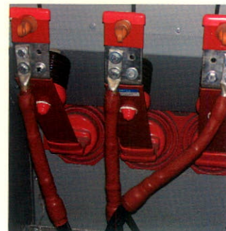
DSG-Canusa 15 kV medium voltage termination kits.
