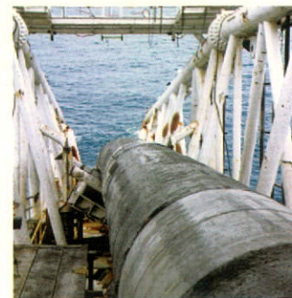
Bredene Shaw Hevicote on world's longest subsea pipeline in the North Sea.
