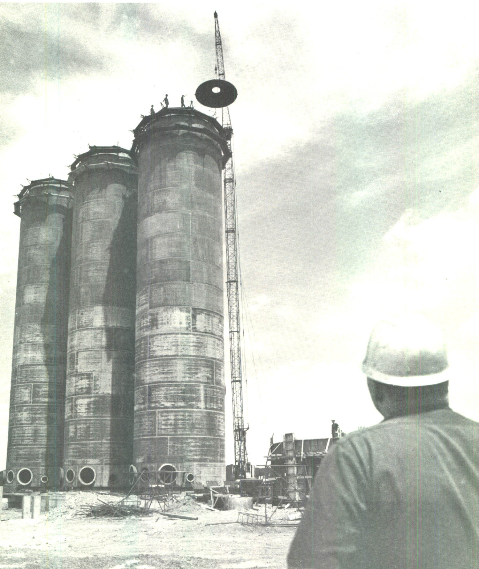
Part of a new steel-making complex in Hamilton, these hot blast stoves – 131 feet tall and 32 feet in diameter – were fabricated and erected by the Plate Fabrication Division.
