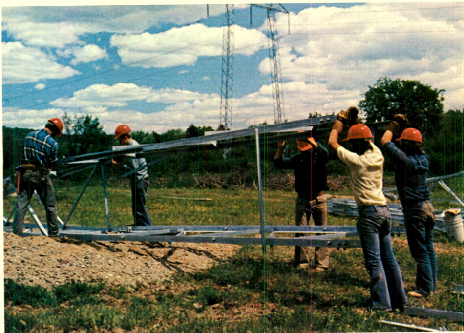
Construction of 345 KV line between Keswick and Coleson Cove. NB Power staff devised unique method of ground assembly of towers and hoist erection.
