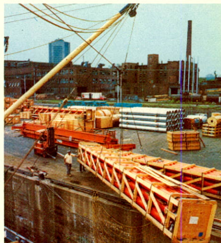
Line pipe destined for above ground use in the Arctic, is jacketed in Stelcolour steel for protection and identification purposes, and shipped from Montreal.
