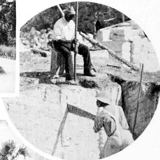
COLORED LABORER IN QUARRY SAWING OUT BLOCKS OF CORAL
