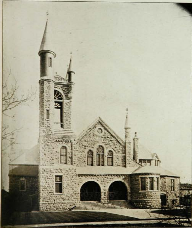
ST. JOHN'S PRESBYTERIAN CHURCH, CORNWALL, ONT.
