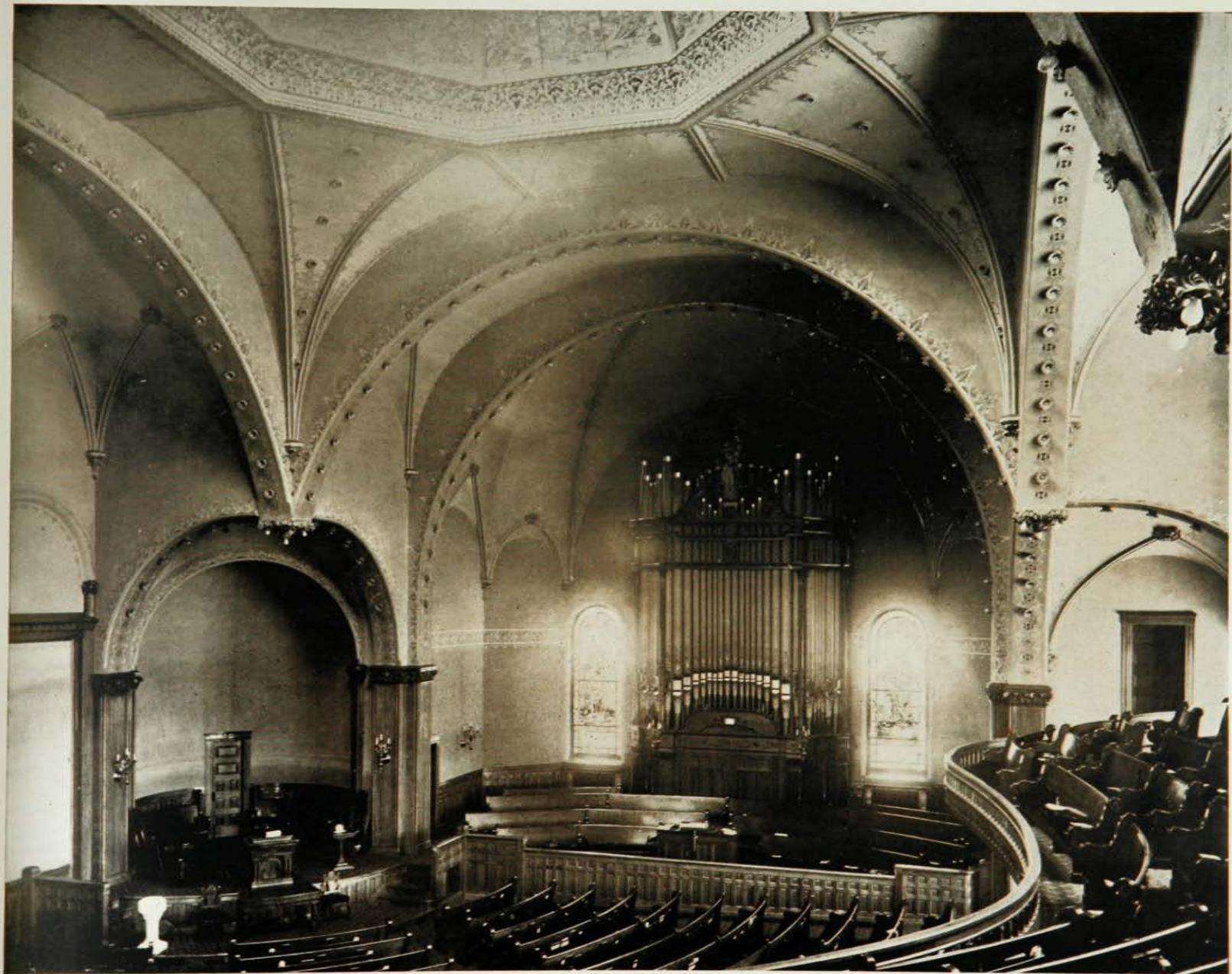
INTERIOR OF PILGRIM CONGREGATIONAL CHURCH, CLEVELAND, O.
