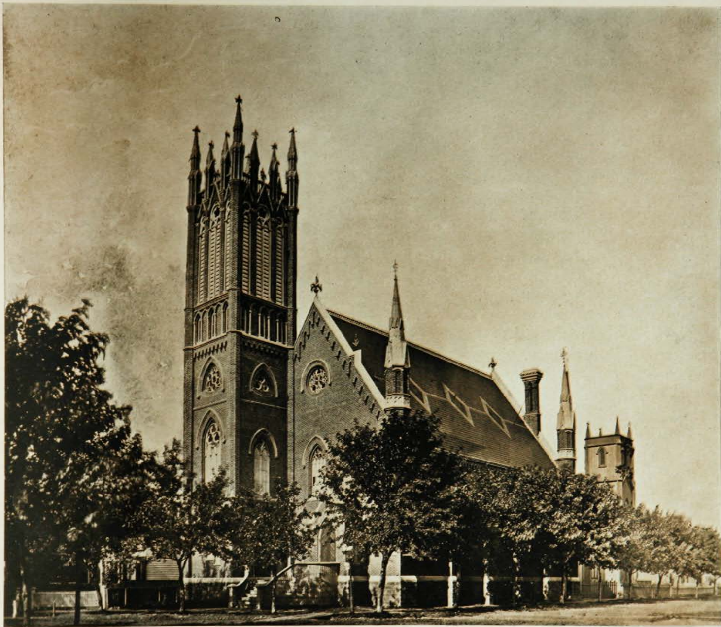
WELLAND AVENUE METHODIST CHURCH, ST. CATHARINES, ONTARIO.
