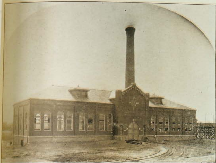
POWER HOUSE, NEWPORT, KY.
