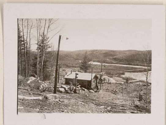
Ski Hill looking down to the Maurice The bridge can be seen left centre and on the far shore the construction road.
