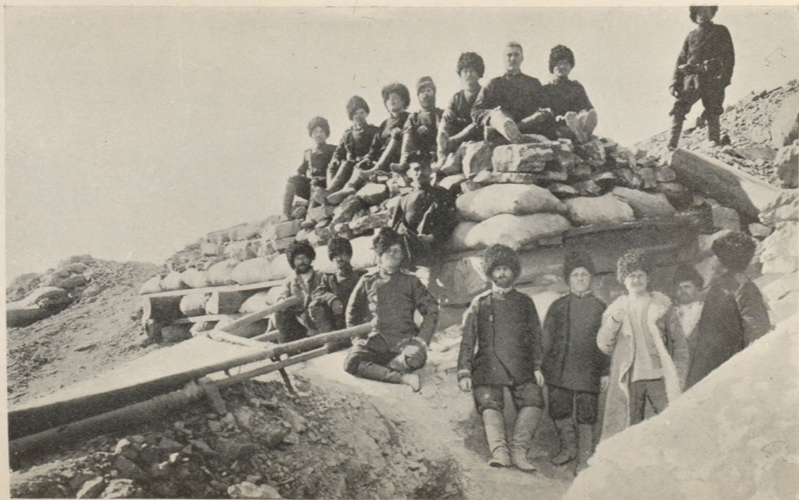
BLINDAGE ON THE LEFT FLANK OF 203 METRE HILL. THE MEN ARE RIFLEMEN OF THE 2ND COMPANY, 5TH REGIMENT.
