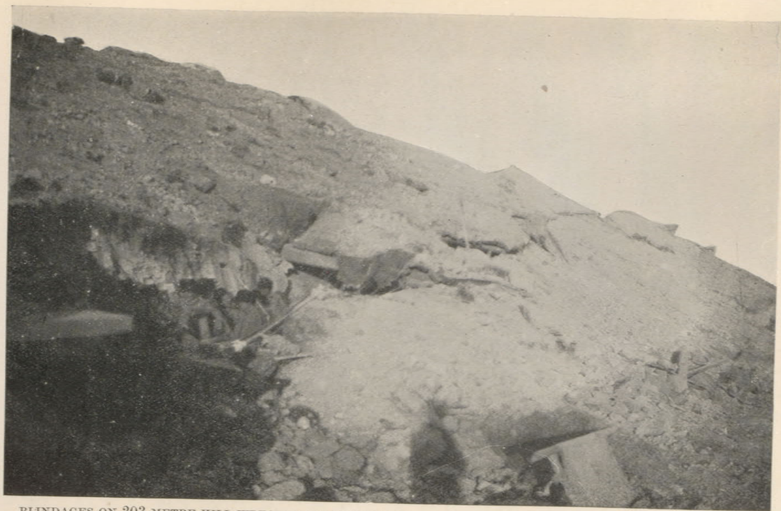
BLINDAGES ON 203 METRE HILL WRECKED BY SHELL FIRE. THE MEN ARE SITTING AMONGST THE RUINS OF A BLINDAGE COMPLETELY DESTROYED BY A 11-INCH SHELL.
