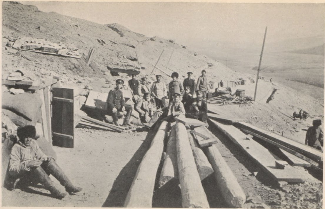
CONSTRUCTING THE ROAD ON THE REVERSE SLOPE OF 203 METRE HILL.
