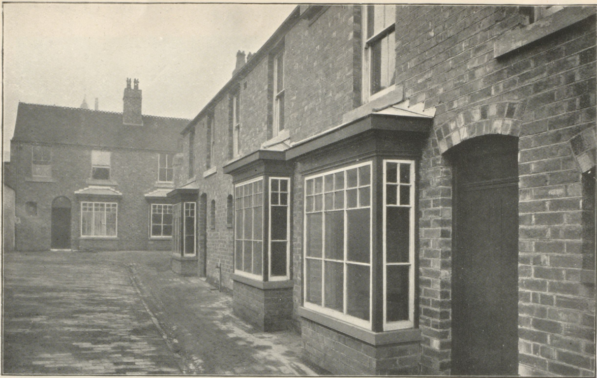
Court, back of 294 Summer Lane. SHOWING HOUSES IN COURT REPAIRED, AND OUTHouses AND OBSTRUCTIVE BUILDINGS REMOVED.
