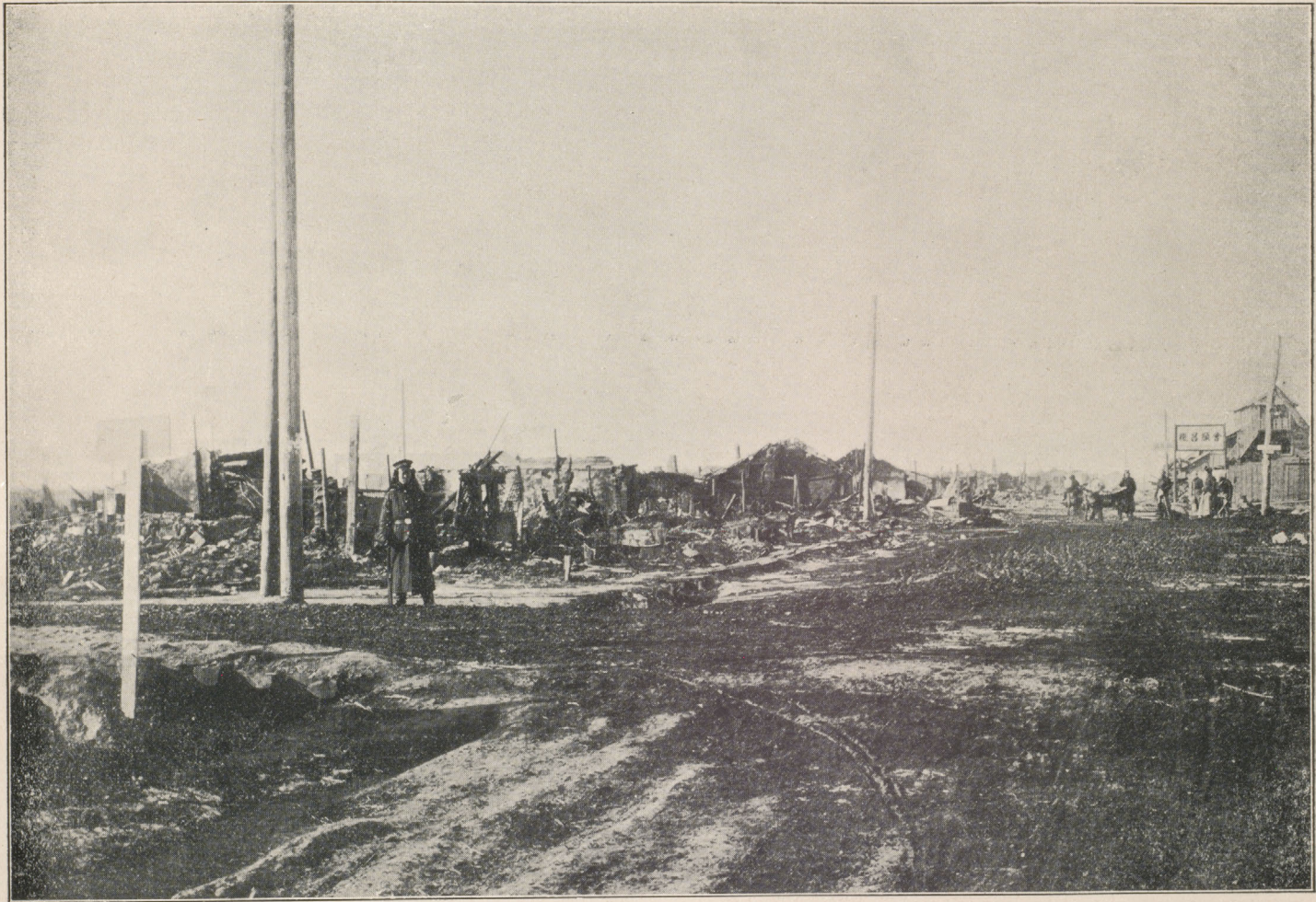
59. Long row of burnt houses.
