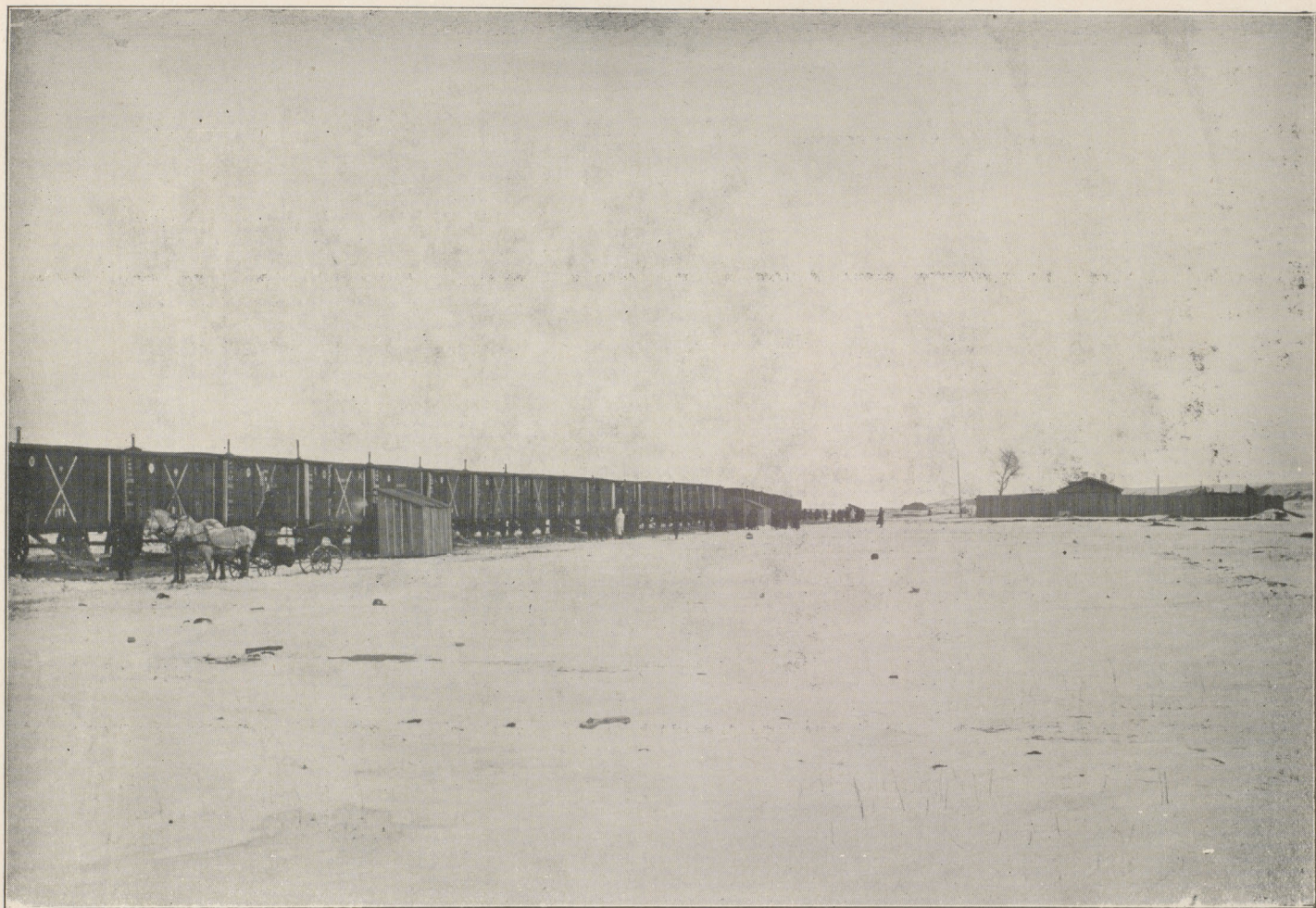
41. The Quarantine Station. Row of 100 railway wagons on left; Suspect Hospital on right.
