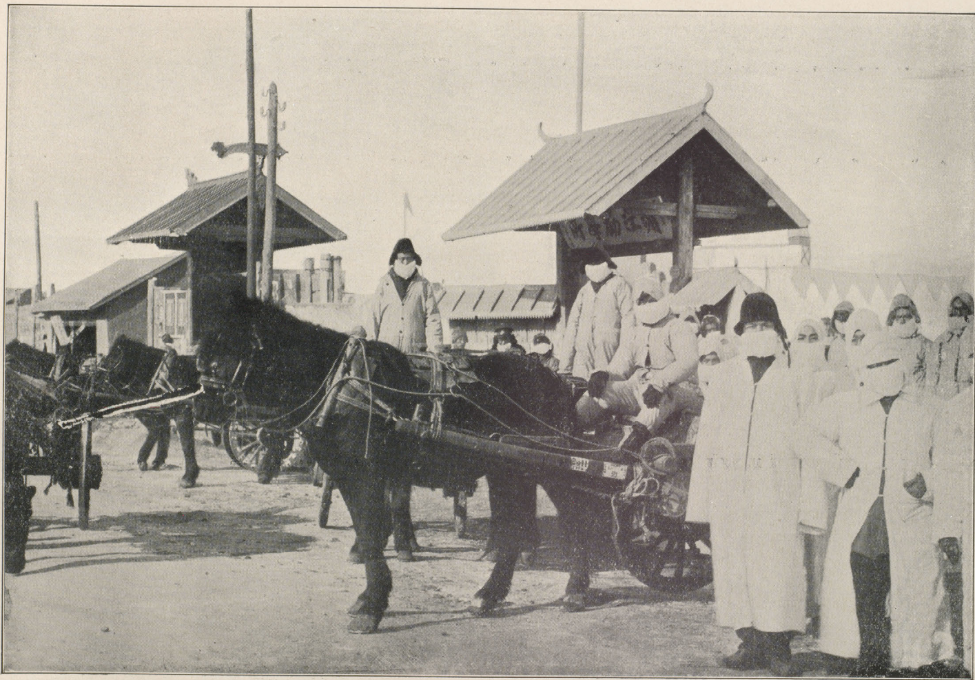
24. Disinfecting carts ready to go out.
