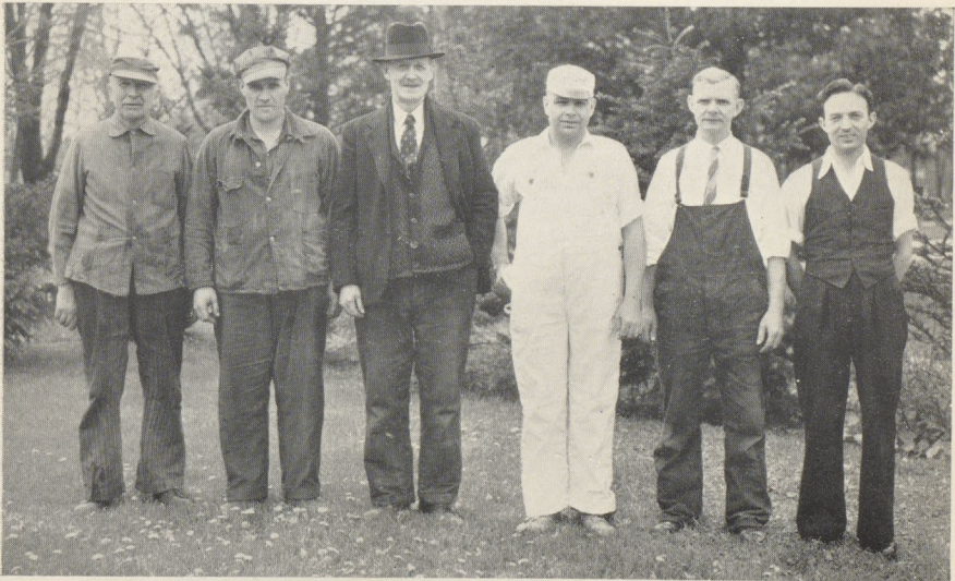
Engineers, Electrician, Painter, Carpenter, etc.
