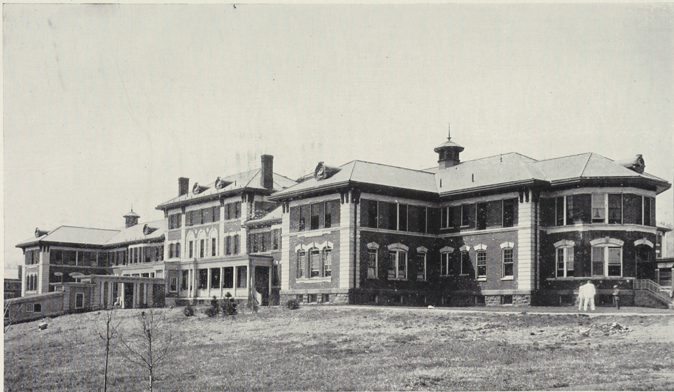
ACUTE HOSPITAL BUILDING—ESSEX COUNTY HOSPITAL FOR INSANE, OVERBROOK, N.J.
