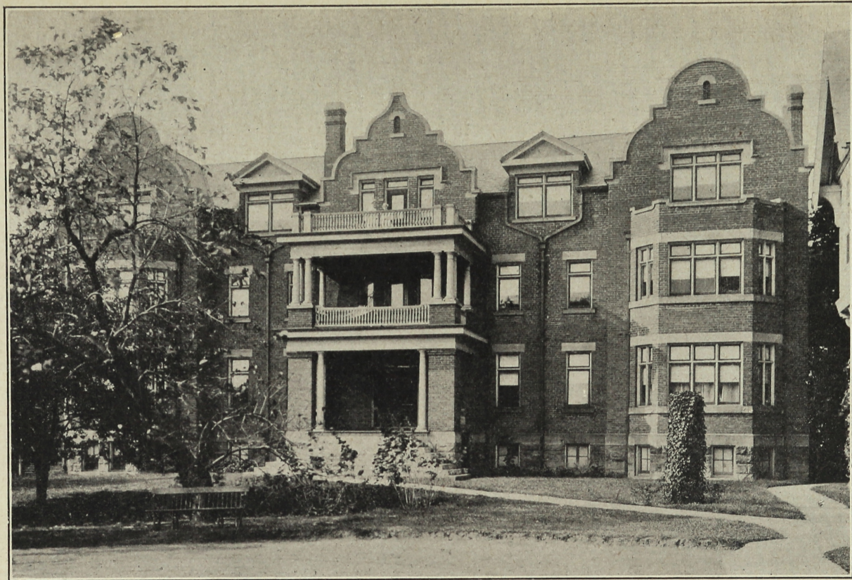
THE NURSES' RESIDENCE, TORONTO HOSPITAL FOR INCURABLES. CORNER STONE LAID BY LADY MORTIMER CLARK, JUNE, 1909. OPENED BY EARL AND COUNTESS GREY, APRIL, 1910.
