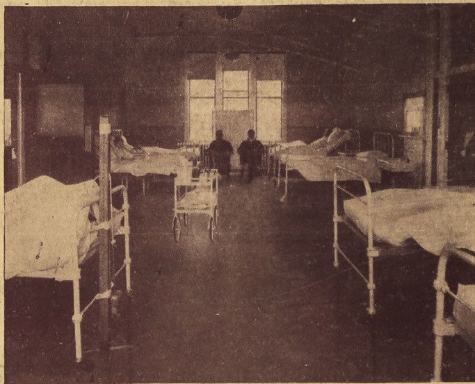
View in St. Joseph's Hospital, Hamilton, Ont. showing Dominion Battleship Linoleum Floor
