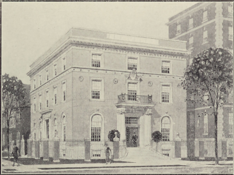
NEW COLLEGE STREET BUILDING, NATIONAL SANITARIUM ASSOCIATION.
