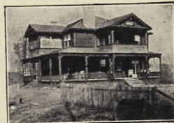
Reception Hospital for Advanced Cases
