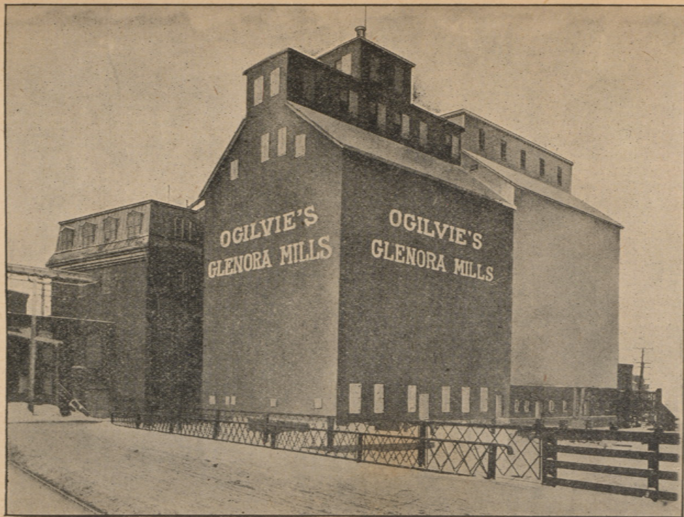
GLENORA MILLS, CAPACITY 2,000 BARRELS FLOUR PER DAY. THE OGILVIE FLOUR MILLS COMPANY, LIMITED, MONTREAL.
