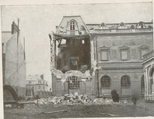
MUSEUM — RIGHT WING OF REAR FAÇADE DAMAGED BY AERIAL TORPEDO IN 1918.
