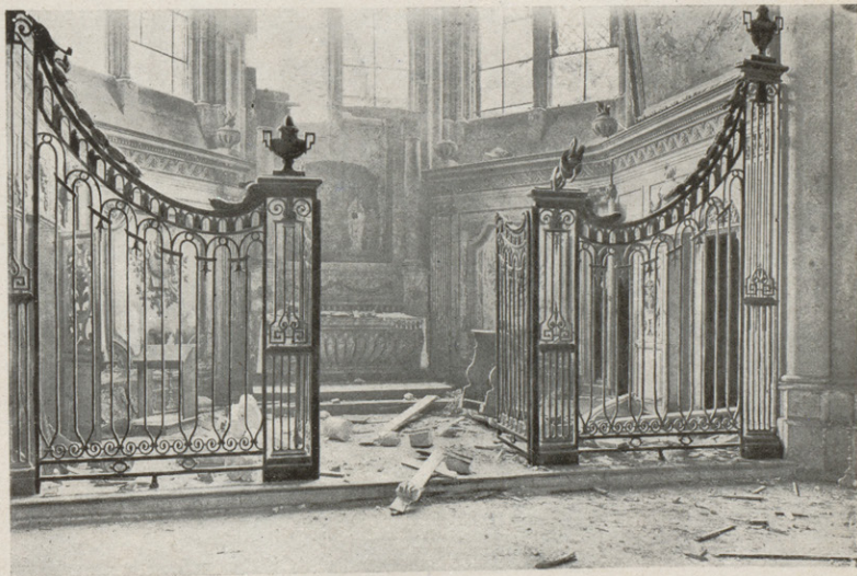
CHAPEL OF ST. JOHN THE BAPTIST DAMAGED BY SHELL. (left-hand side of Apse)
