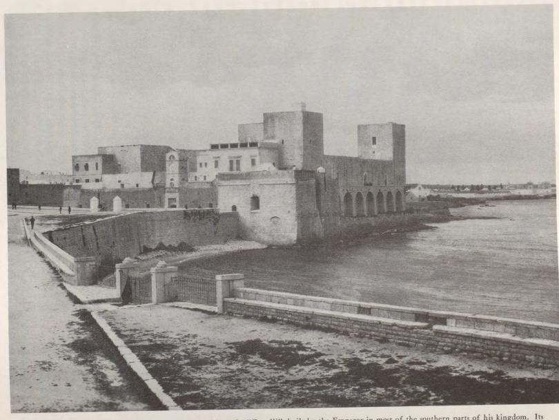
PLATE 130.—Castel Trani, now a prison. It is typical of the "Castelli" built by the Emperor in most of the southern parts of his kingdom. Its walls facing the sea are twenty-seven feet in thickness.
