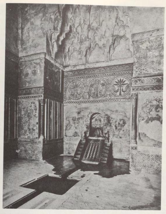
PLATE 185.—Vestibule of the Palace of La Zisa, Palermo, built by William I, showing the characteristic Saracenic stalactite vaulting, mosaic frieze with palms, peacocks, and bowmen. A further Arabic touch is the wall fountain flowing from beneath the Imperial eagle over a marble inclined plane carved geometrically to produce a sense of volume and to increase the apparent rippling of the water.
