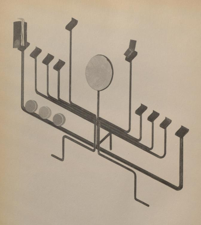
Perfumery display fixture of brass pipes with blue mirror in the center. The adjustable shelving makes it adaptable to small and large quantities of merchandise. FREDERICK KIESLER, architect (New York)
