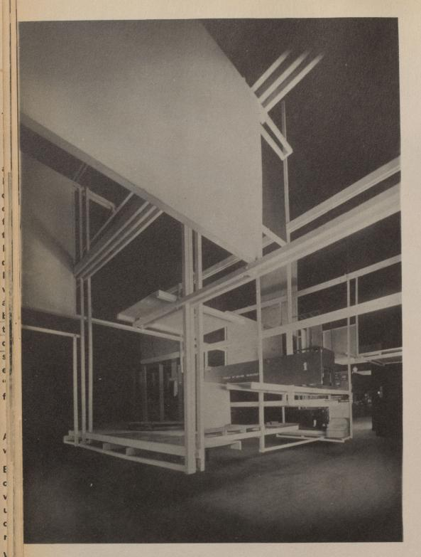
Model of a whole city in which houses, streets, landing stages, etc., are spanned and suspended above each other and next to each other in space. First example of "tensionism," an elastic building system of tubes, platforms and cables, developed from bridge building.
