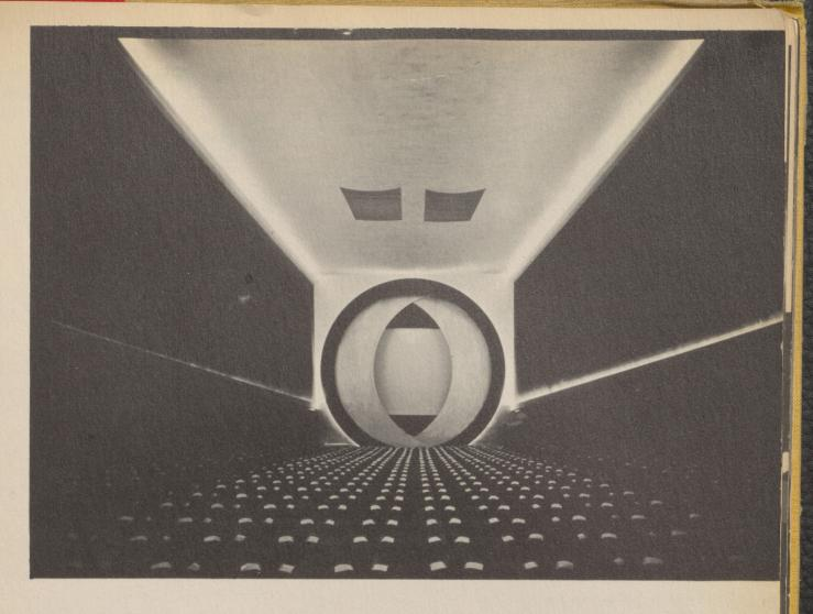
To concentrate the public's attention on the screen moving diaphragms were installed in front of it. These were called the "screenoscope." The diaphragms give to the curved screen behind them any shape and size.
