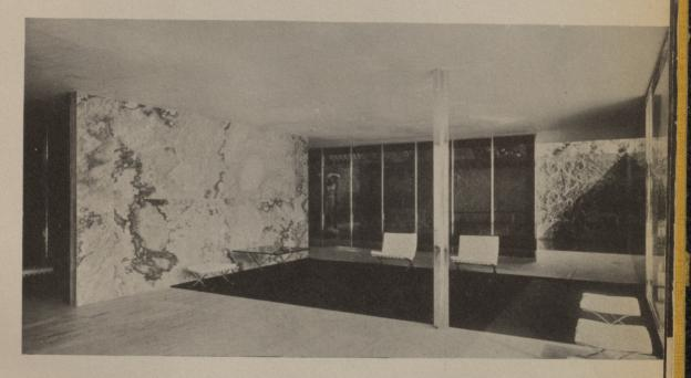
There is no distinction between interior and exterior in contemporary architecture. One material provides both the inner and outer sides of the walls. The natural beauty of the nickel plated steel columns, as well as the marble and glass of the walls, used in
