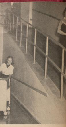
Ramps provide connection between the different floor levels of the two buildings.
