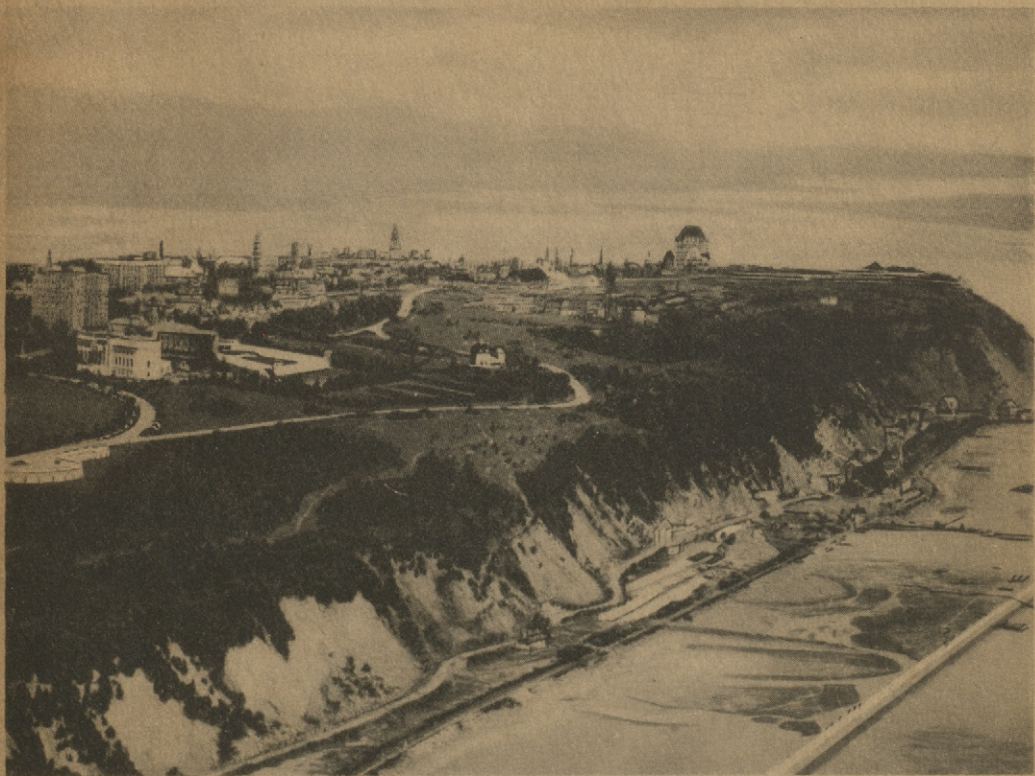
QUEBEC AND ITS SETTING FROM THE WEST
