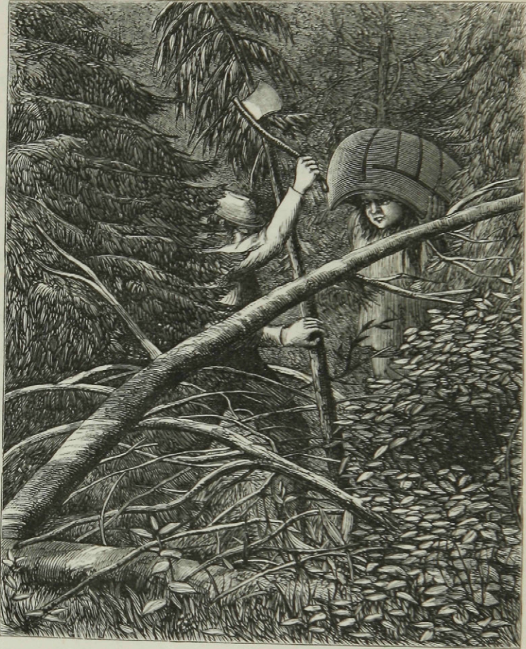
CUTTING OUT A ROAD.
