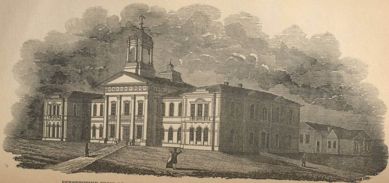
PERSPECTIVE VIEW OF THE NEW NORMAL SCHOOL AND EDUCATION OFFICES FOR UPPER CANADA.
