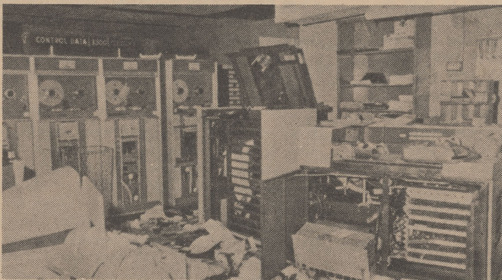
Wrecked Control Data Installation
