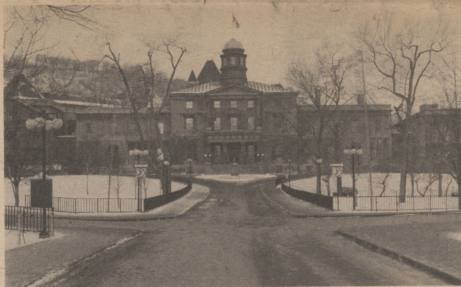
Above and below: The McGill Arts Building circa 1860 and today.
