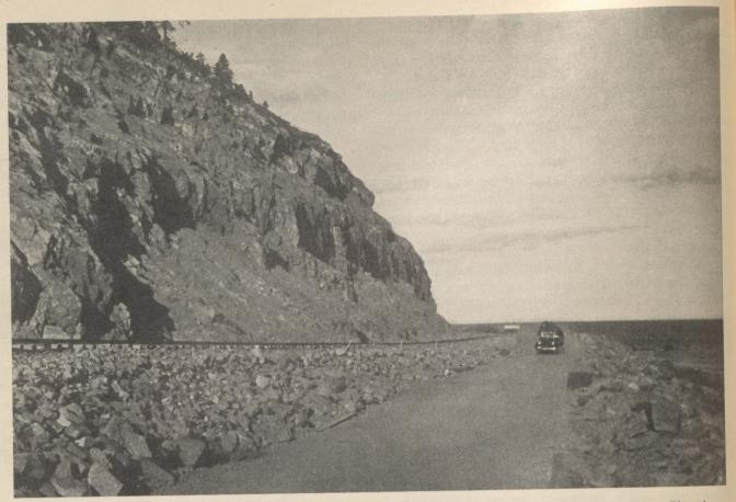
First task in the construction of the town of Baie Comeau was the building of a road from the docks to the townsite. Blasted out of solid rock which stretched down to the water's edge, this modern highway and railroad make transportation possible.
