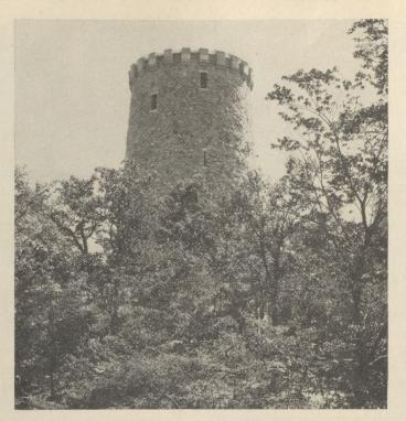
The water and observation tower, standing on the highest point of the island, is ninety-six feet in height and thirty-six feet in diameter at the top.
