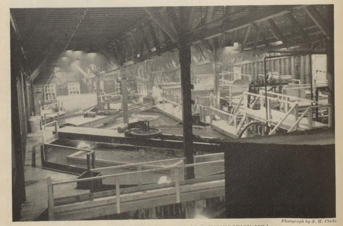
GENERAL VIEW OF THE INTERIOR OF A CYANIDATION MILL Two thickeners at left, agitators at right, filter in left background.
