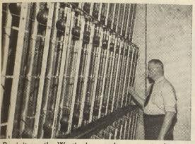
Precipitron, the Westinghouse electronic air cleaner, removes particles as small as 1/250,000 of an inch.
