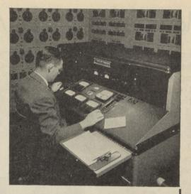
A.C. CALCULATING BOARD Saves thousands of dollars by providing rapid solutions of the complex electrical problems of ever expanding power systems.
