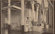
Stoker Fired Cross Drum Boiler
