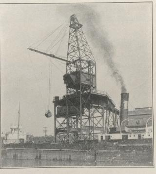
Portion of coal and coke handling plant on Lachine Canal built for Montreal Light, Heat & Power Co. Capacity of tower 300 tons an hour. Storage capacity 250,000 tons.
